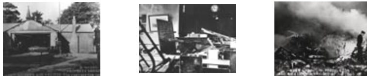
The Aftermath: left and centre, the school and right, the Snack Bar.
